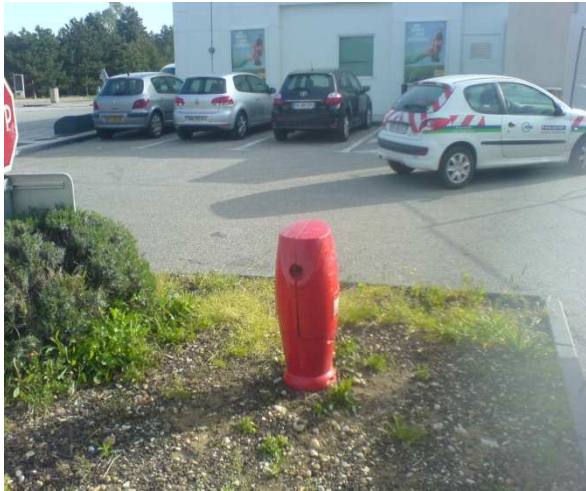
Poteau incendie aire ouest- nord station service
